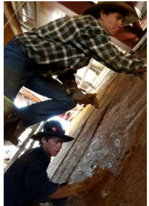
Bob and Harry Elliott hard at work rendering the concrete walls
